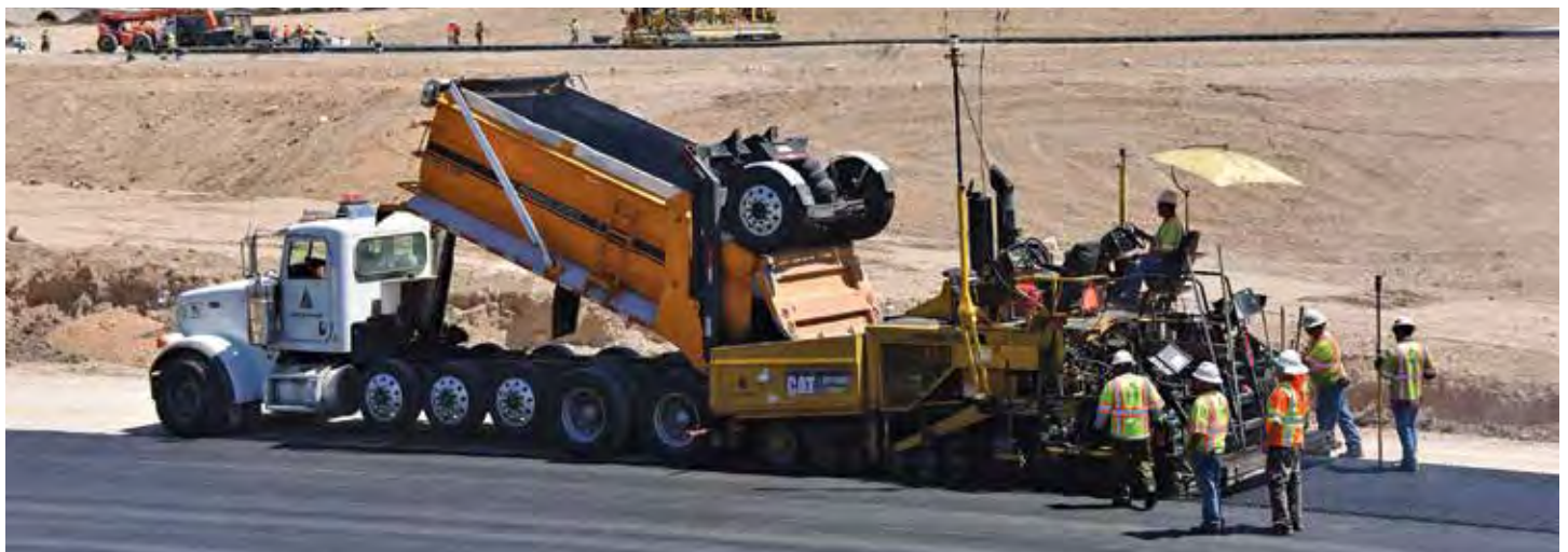
(photos courtesy Staker Parson Cos.)
